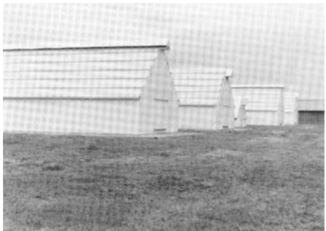
Fig. 1. Warehouses used in study, left to right, (1) naturally ventilated, 8% m.c.; (2) mechanically ventilated, 8% m.c.; (3) not used; (4) naturally ventilated, 10% m.c.; and (5) mechanically ventilated, 10% m.c.
